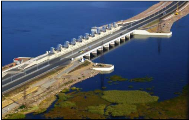
Figure 6 – St. Petersburg Barrier sluice gates
