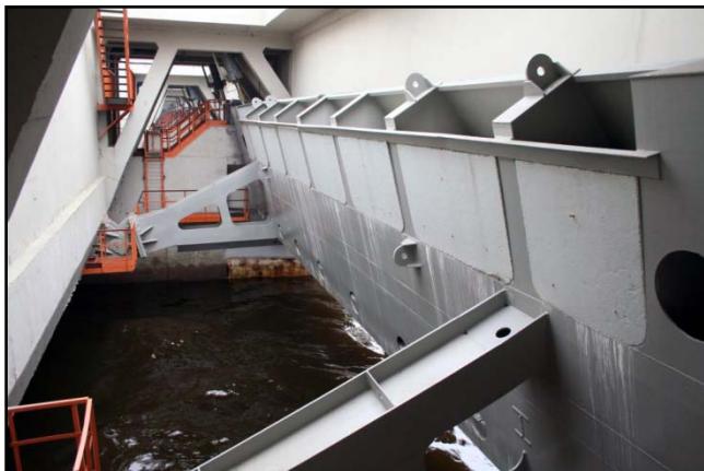
Figure 10 – St. Petersburg sluice gate inside housing
