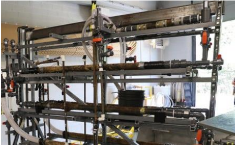
Corrosion Control Evaluation Studies
