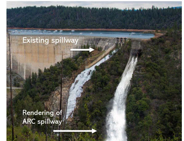
New Bullards Bar Dam Atmospheric River Control spillway Source: Yuba Water Agency
