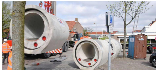
In-pipe heat recovery, applied with new installation or replacing sewers (Courtesy: Rabtherm)
