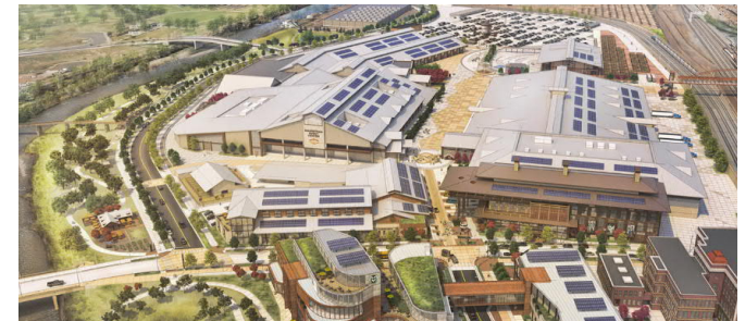
Architectural rendering for National Western Center (Denver, CO) – 3.8 MW sewer thermal DES under construction
