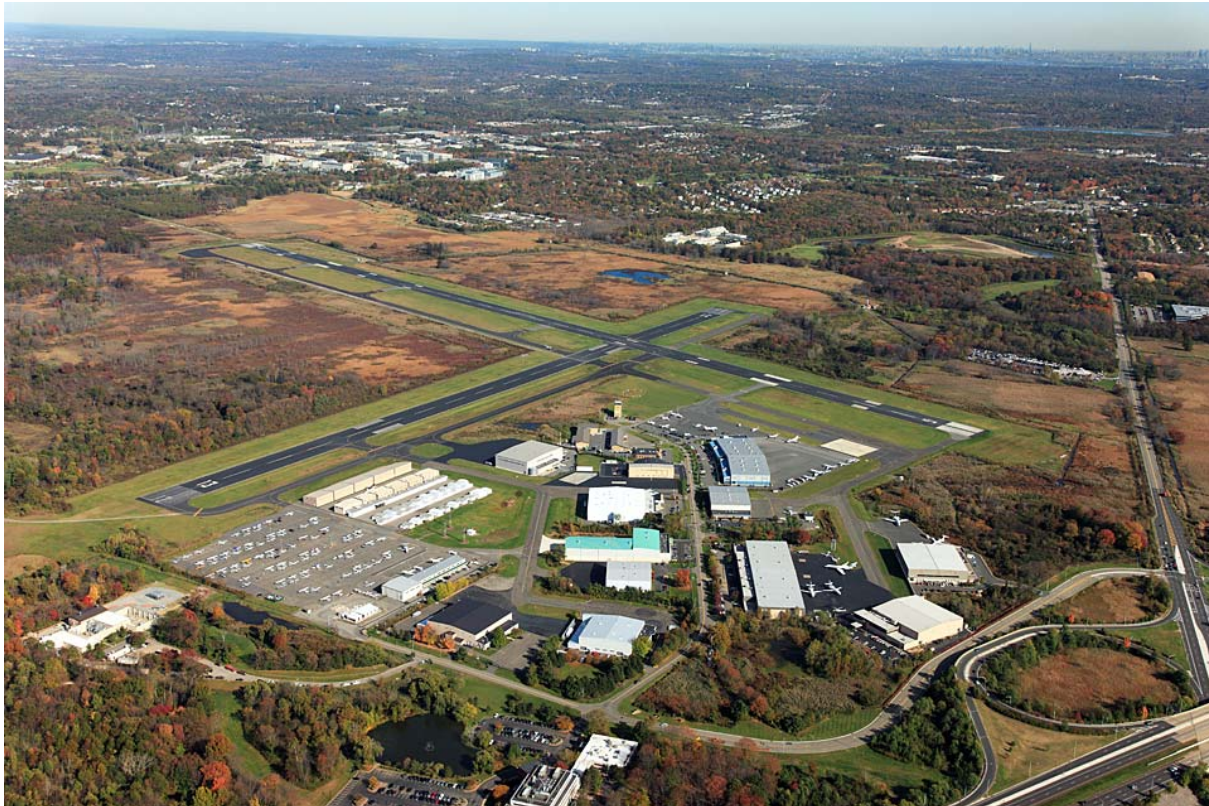
Figure H.6. Morristown Municipal Airport
