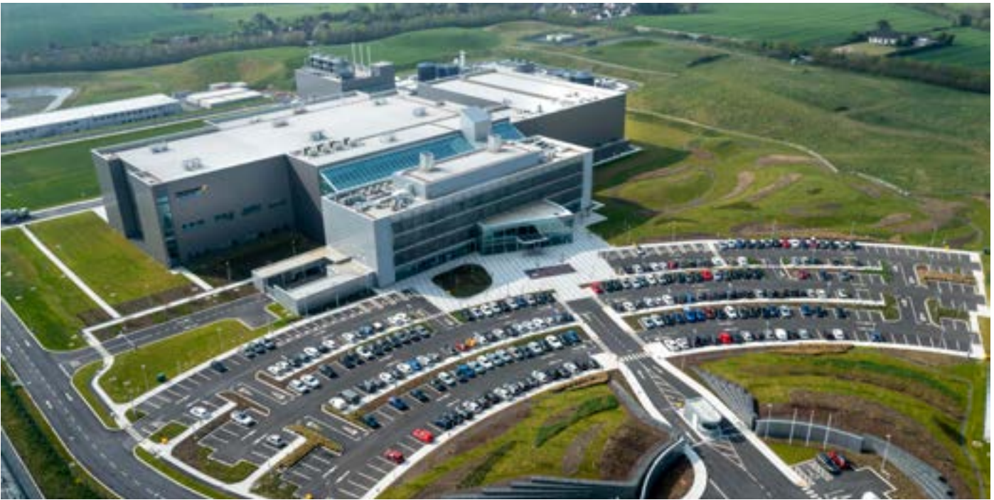
WuXi Biologics Drug Substance Manufacturing Facility
